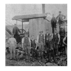
last week fixed into position on top of the guarry and used for the first time here on Tuesday, when everything appeared to be in perfect order. The boiler, which was of 10-horse power, forced the steam through pipes to the bottom of the quarry, a distance of some 60 or 70 feet, where the machinery which pumped the water to the top was situated. It was therefore attached to no engine on the bank.
